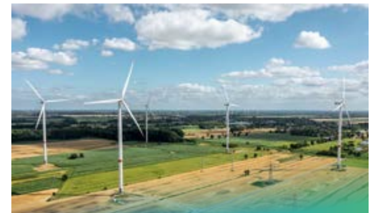
CC4E's Curslack Research Wind Farm, approx. 1 km from the Energy Campus Technology Center
