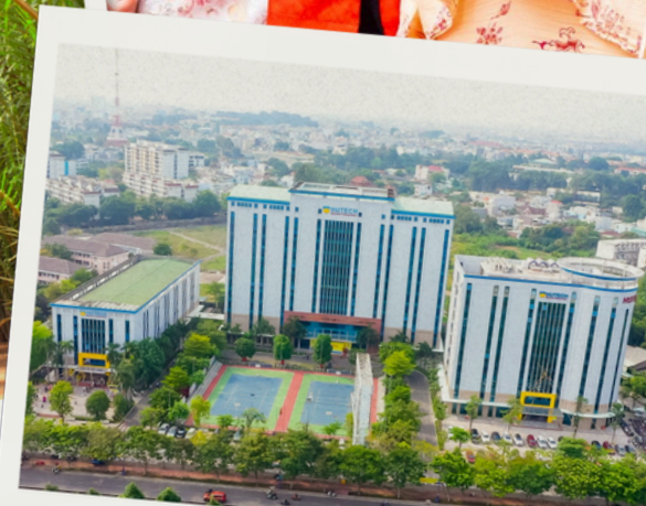
HUTECH Hi-Tech Park Campus
